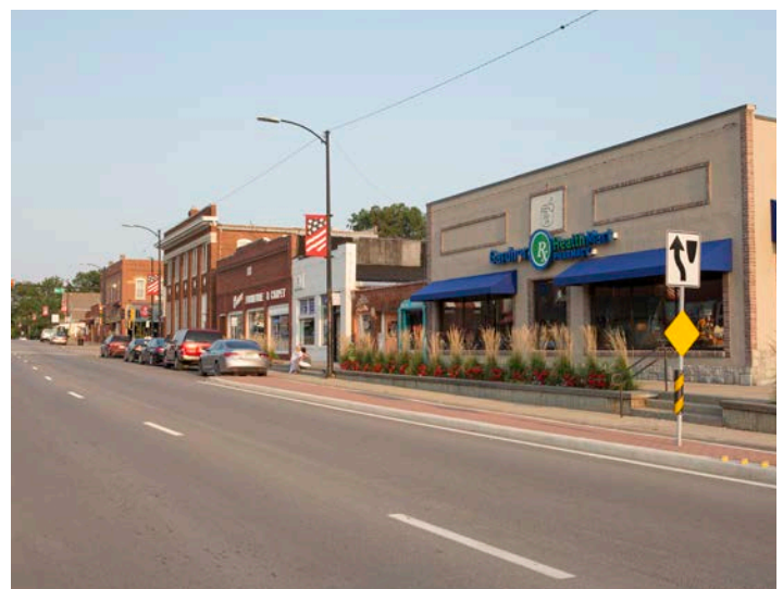
Figure 1.02 - Businesses along Main Street
