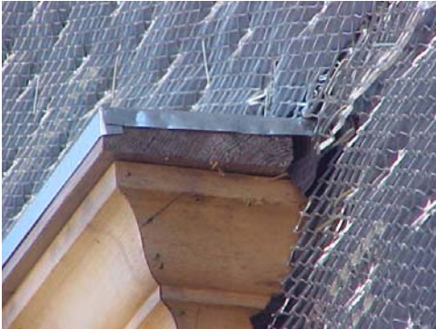
Flashing (drip cap) should be bent down over the end of the trim boards to prevent water infiltration under the flashing
