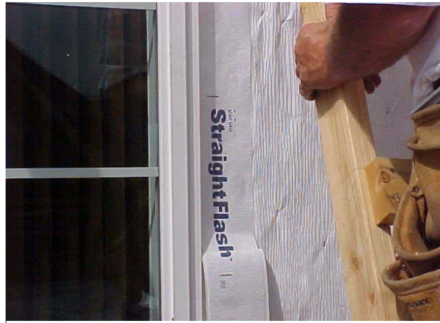
Side jamb flashing tape installed shingle style
