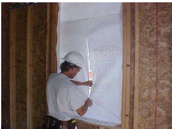
Making the modified "I" cut in housewrap — a straight "I" cut is also acceptable
