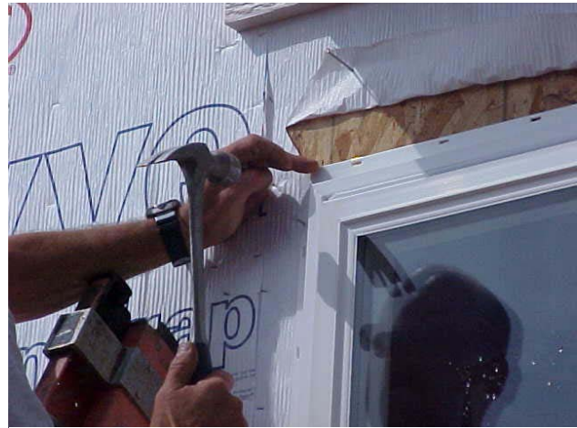
Fasten in place with galvanized roofing nails
