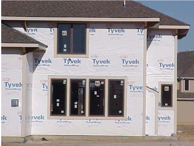
Continuous drainage plane over entire building
