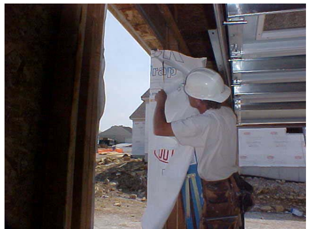
Bring housewrap back to the inside wall
