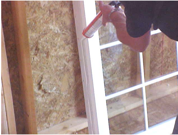
Apply a 3/8" bead of sealant up each side and across the top of the nailing flanges
