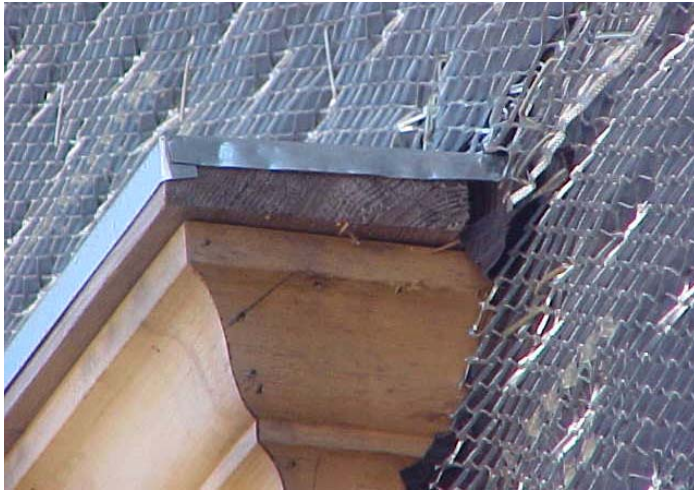
Flashing (drip cap) should be bent down over the end of the trim boards to prevent water infiltration under the flashing
