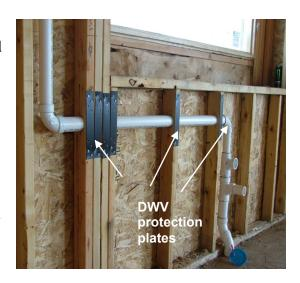
drain and vent piping may be ABS plastic, polyvinyl chloride (PVC-Type DWV) and other materials as listed in the code. Above ground sanitary drains and vent piping may be ABS plastic, polyvinyl chloride (PVC-Type DWV) and other materials as listed in the code. All piping materials shall be labeled with the manufacturer's mark or name and the quality or grade of the product.
