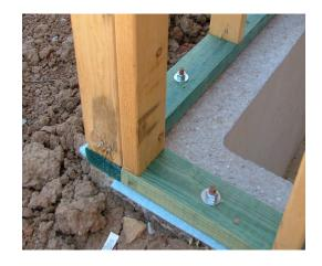
\* Before framing, find and seal all water and air infiltration/penetrations spots around the basement where accessible. This will greatly help to avoid heat loss and insect intrusion.
