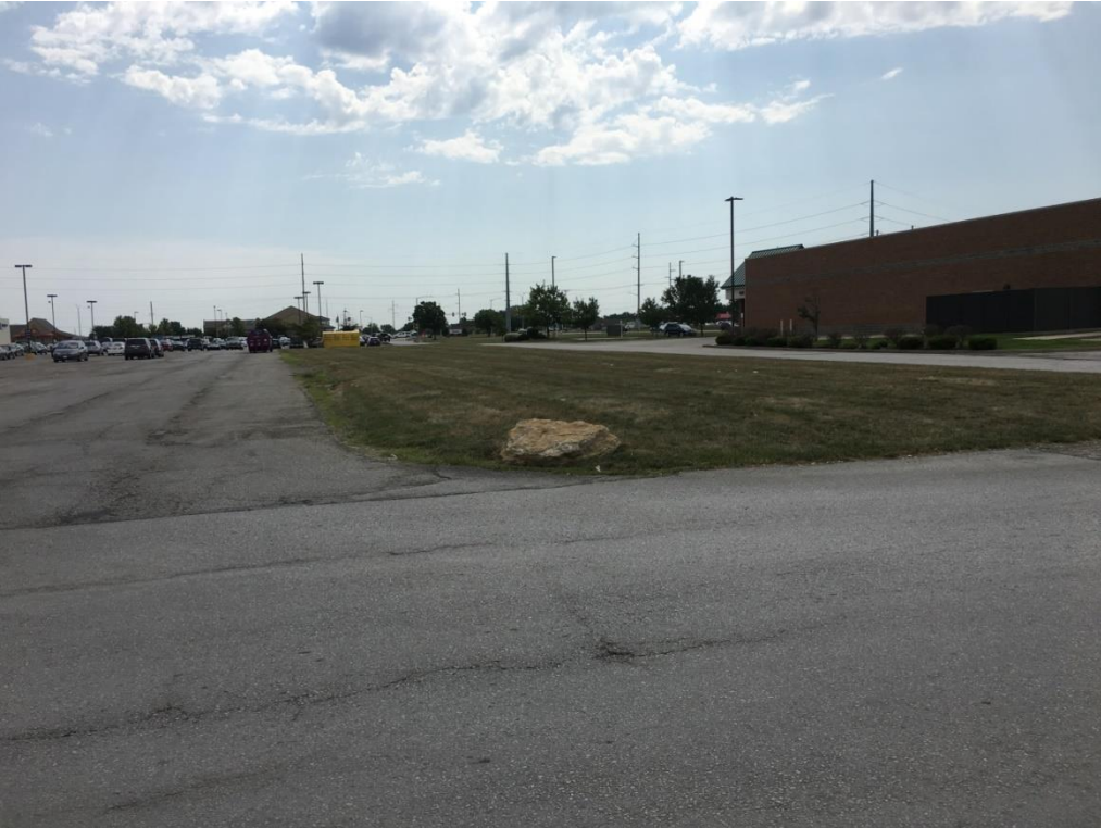
Photograph 22- Private Drive Looking East into the Redevelopment District, shown inadequate curbs and infrastructure.
