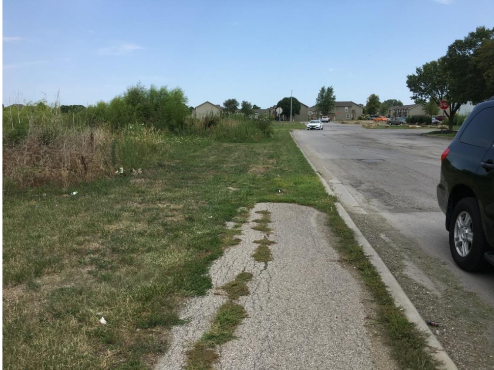
Photograph 17- North South Private Drive, connecting East Main Street to Lincoln Lane Redevelopment District, shown inadequate or crumbling sidewalk.
