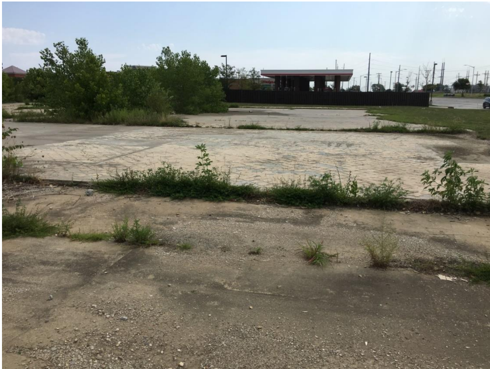
Photograph 13- Existing foundation of two buildings on Lot 2 of the Redevelopment District.
