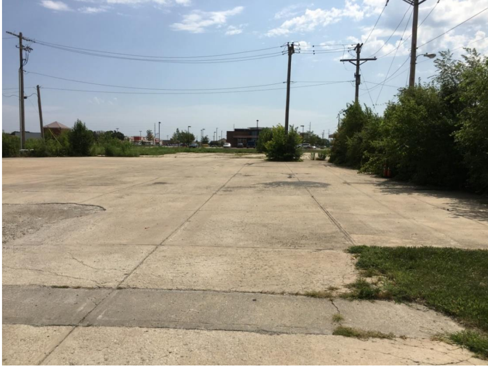
Photograph 14- Existing foundation of two buildings on Lot 2 of the Redevelopment District.
