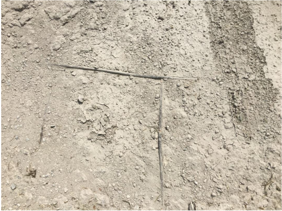
Photograph 15- Existing foundation of two buildings on Lot 2 of the Redevelopment District.
