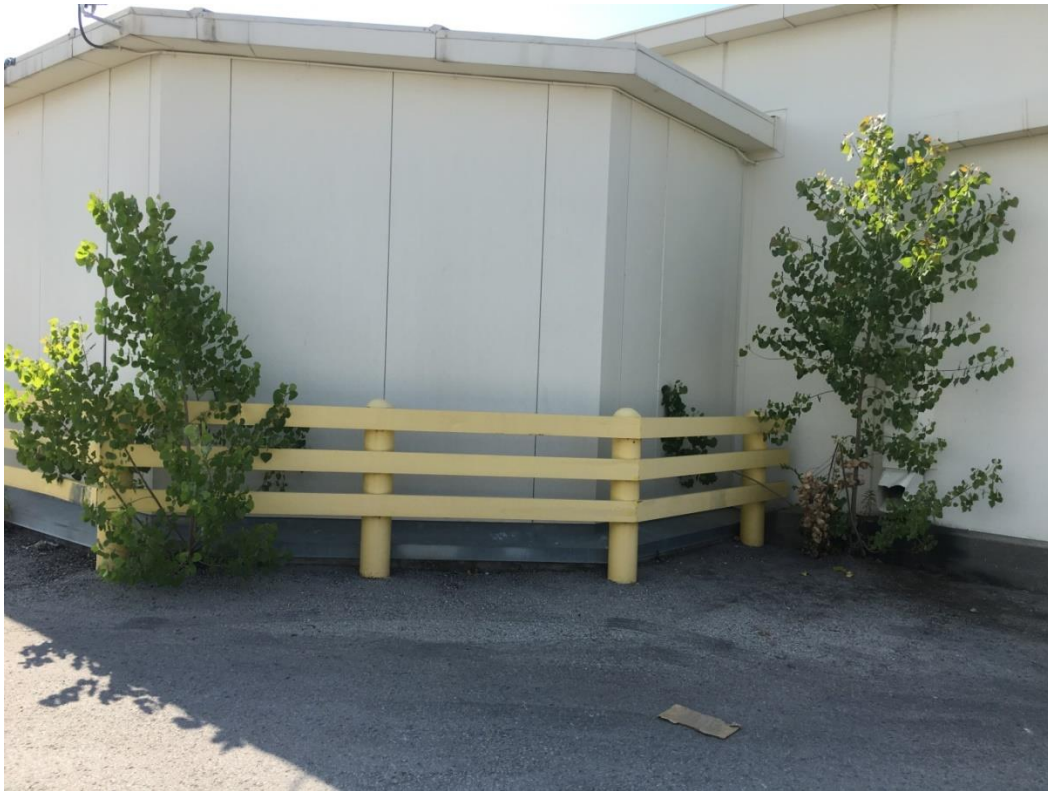
Photograph 40- Location Lot 5- Trees growing at side of building.
