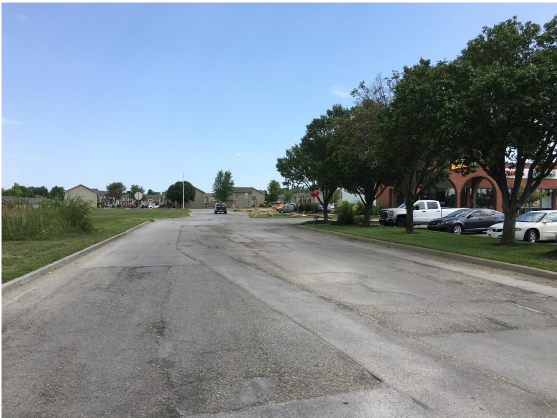
Photograph 16- North South Private Drive, connecting East Main Street to Lincoln Lane Redevelopment District.
