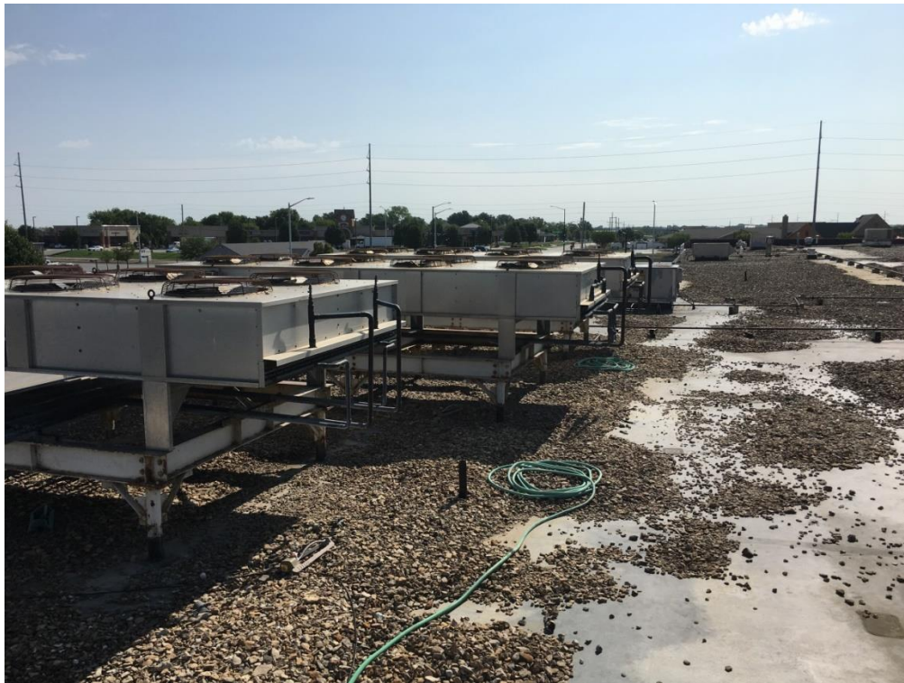
Photograph 2- Roof of 830 E Main Street, single-ply EPDM, rubber-based membranes with gravel top coat. While the age of the roof is unknown, there were many patches.
