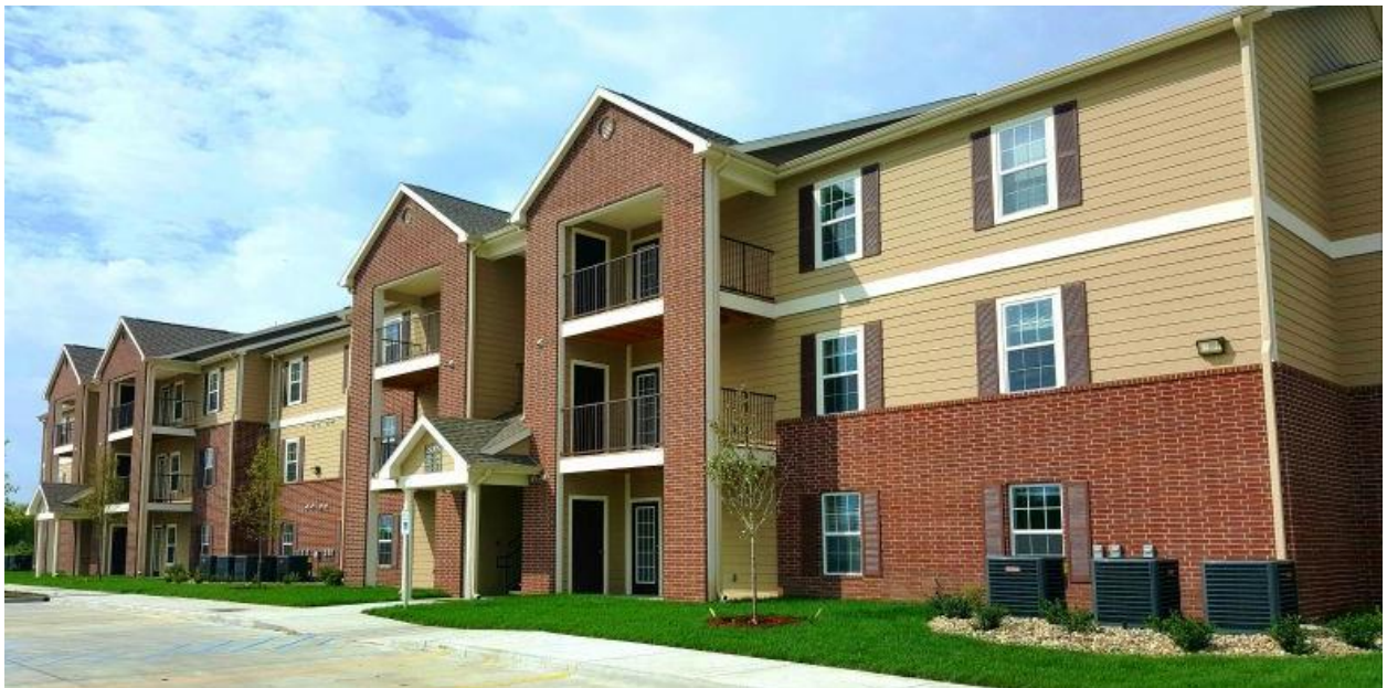
Figure 36 Recent Multi-Family Development in Gardner – Nottingham Village
