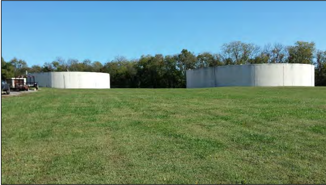
Figure A8: Contact Basin/ First Clearwell (Left) and Second Clearwell (Right) (Facing N), 10/07/2016
