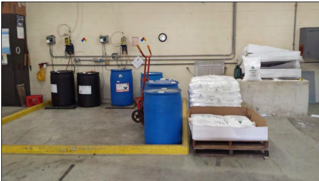
Figure A18: Chemical Storage, 10/07/2016
