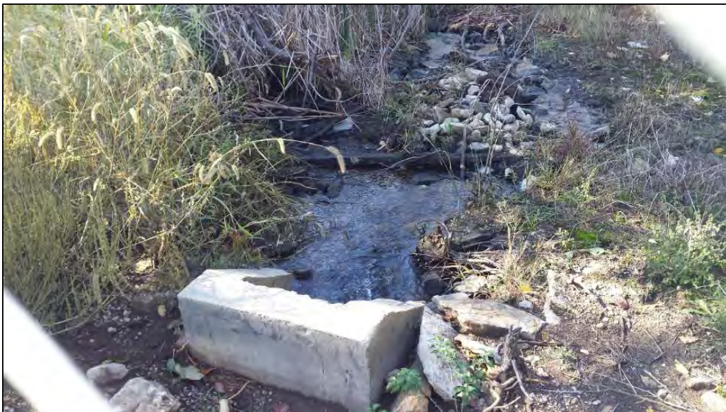
Figure A17: Decant Drain to Surface (South Edge of Property) (Facing S), 10/07/2016
