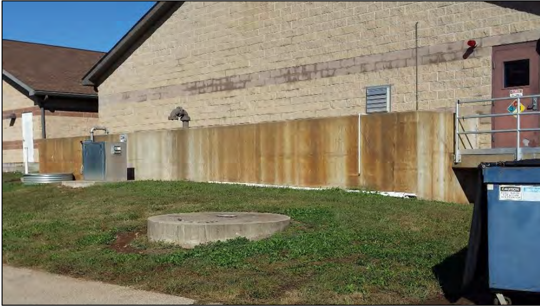
Figure A1: Pre-treatment Basin (Facing NW), 10/07/2016
