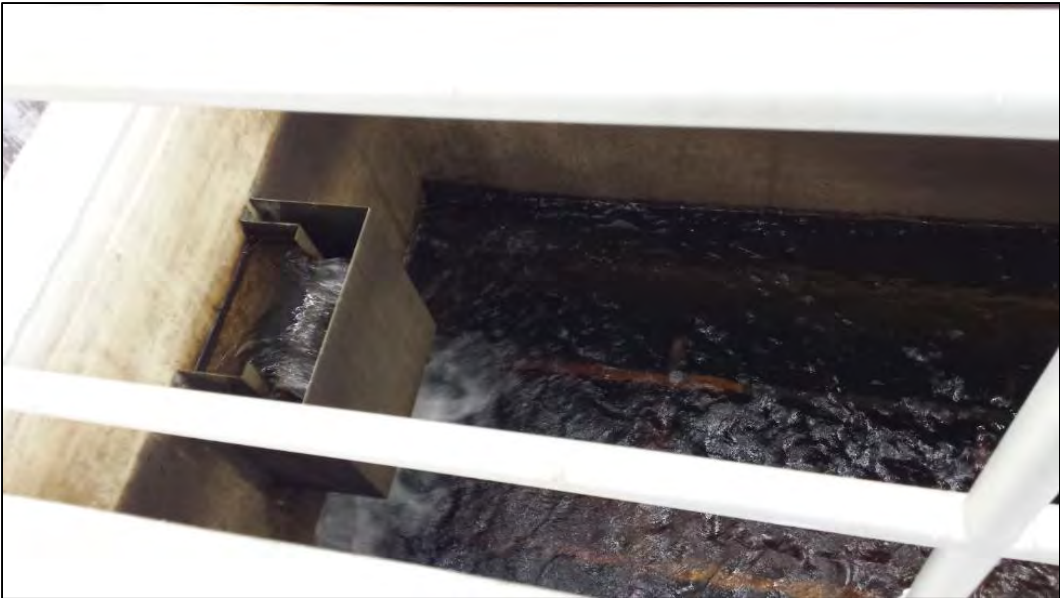
Figure A4: Filter Cells and Splitter Weirs, 10/07/2016
