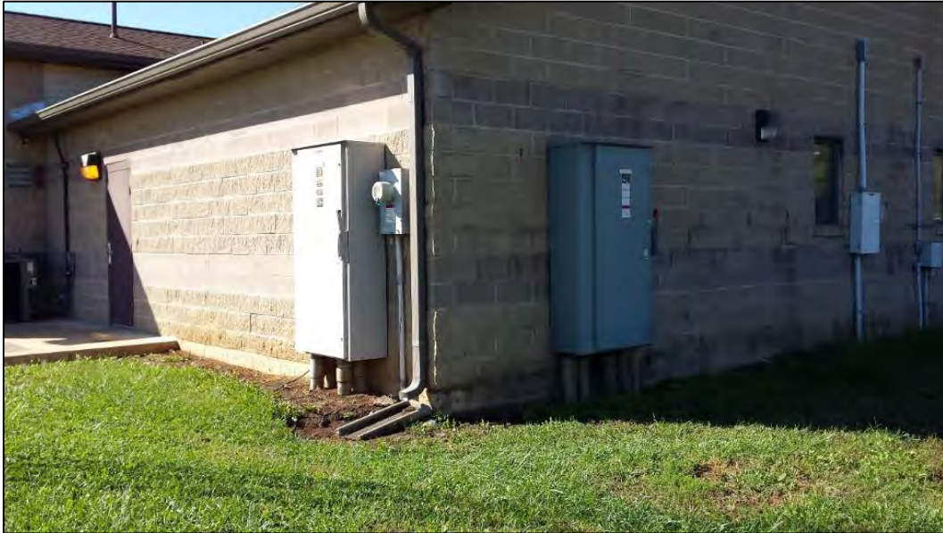
Figure A24: Electrical Boxes on Northeast Corner of Building, 10/07/2016
