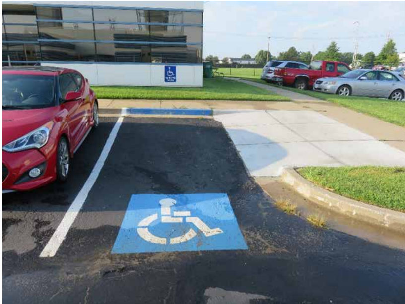
Parking space running slope is excessive (1:48 maximum)
