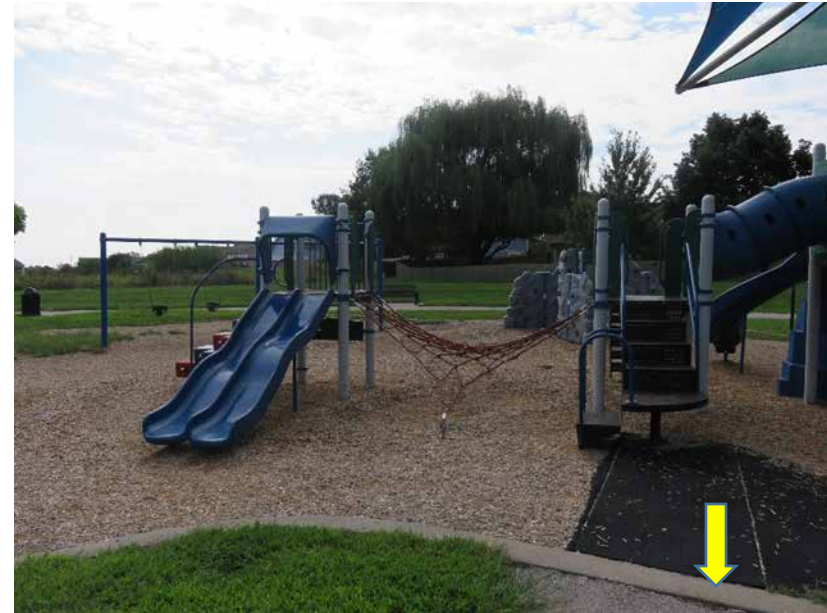
Ground level transition location – mitigate 1-1/2-inch change in level
