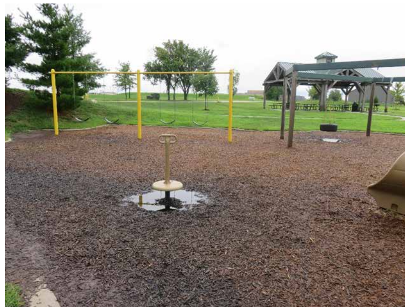
Current inaccessible surfaces are unusable in inclement weather
