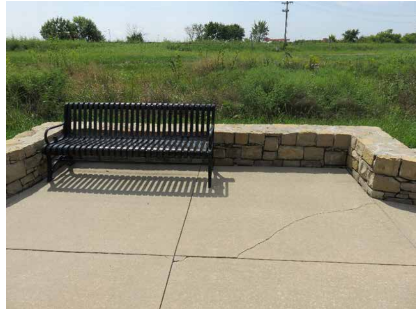
Excellent use of space to provide accessibility to all users.
