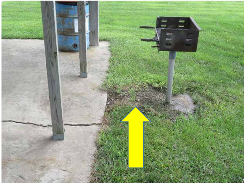
Example of BBQ that can be provided on accessible route Solutions are moving BBQ or installing small firm ground surface
