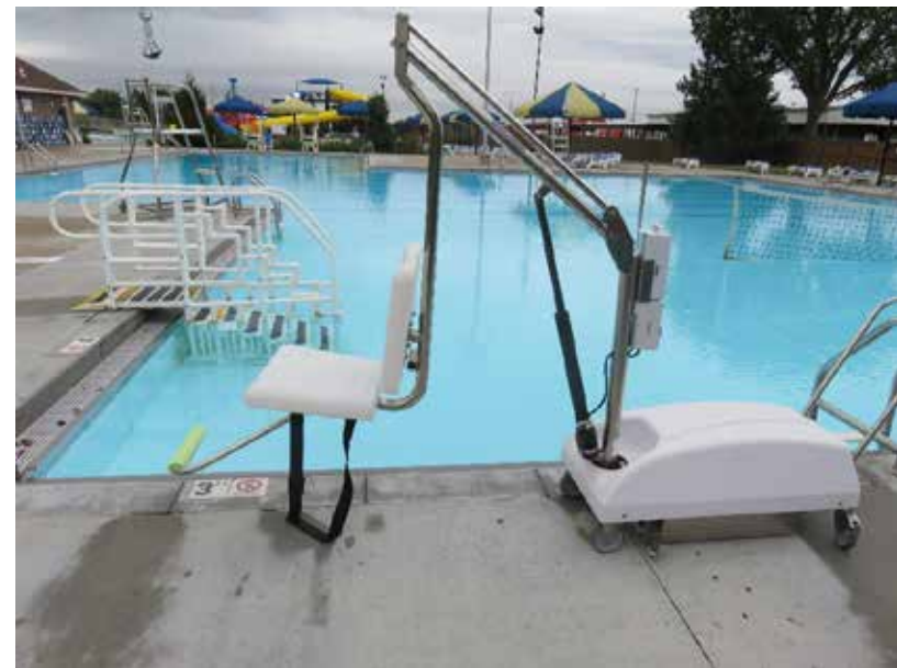
Pool lift not independently operable
