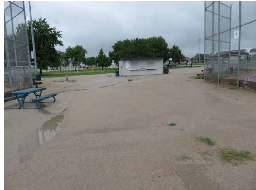
Accessible routes to facility areas compromised in inclement weather
