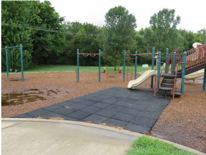
Rubber mats providing route to base of composite play structure
