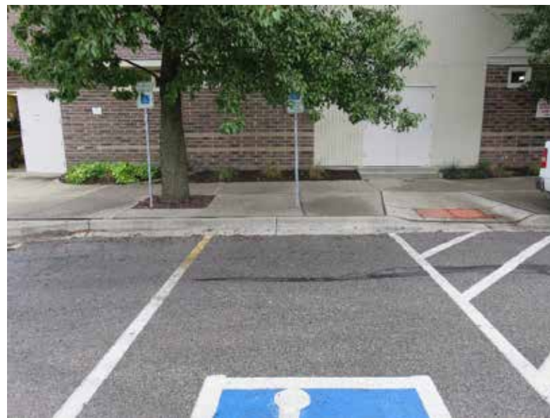
Trim trees to ensure signs are visible
