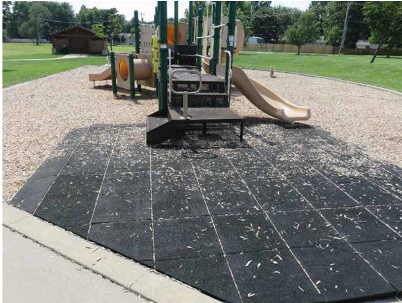
Existing rubber pad surface providing access to base of structure
