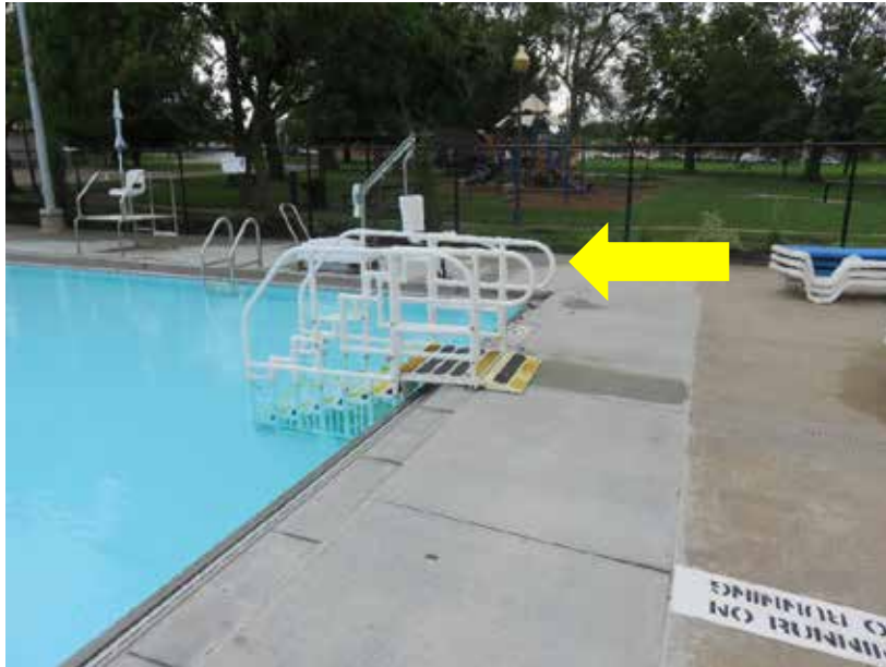
Pool stairs meet many requirements of ADAAG but are unstable
