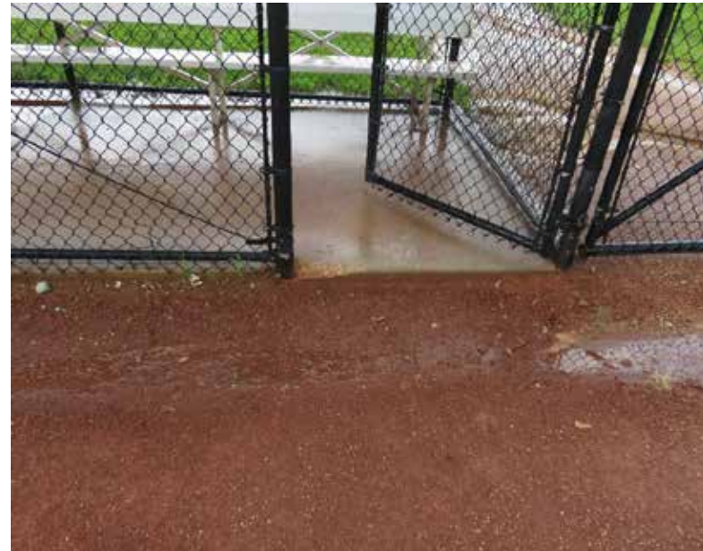
Example of change in level from dugout to field Conditions fluctuate; include in maintenance procedures
