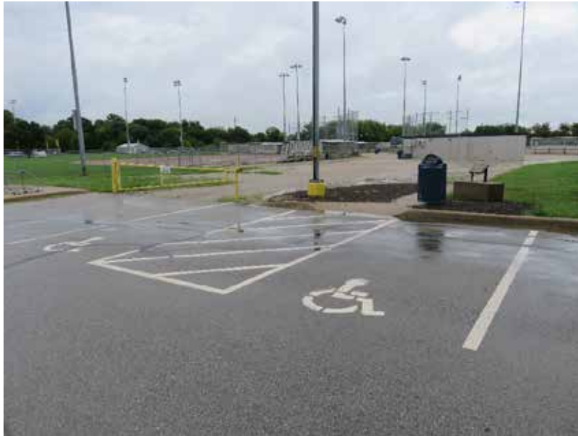
Existing parking needs signage
