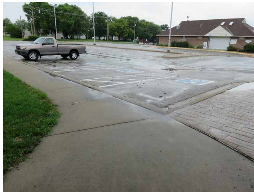
Install compliant curb ramp on an accessible route from parking Position curb ramp to ensure level landing area at top
