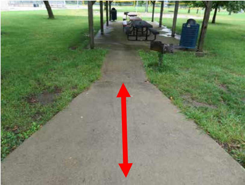
Slope is excessive (12%); regrading and/or ramping needed
