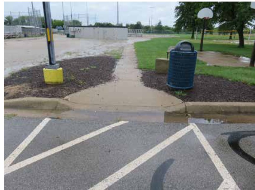
Primary accessible route from parking to facility features
