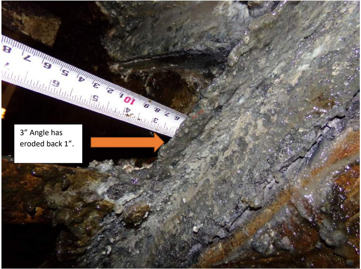
3" Angle has eroded back 1".
