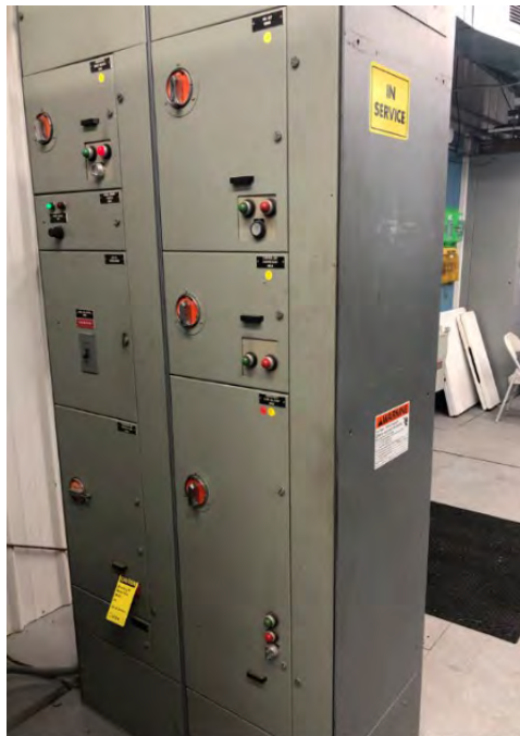
Motor Control Center # 1 Rear View
